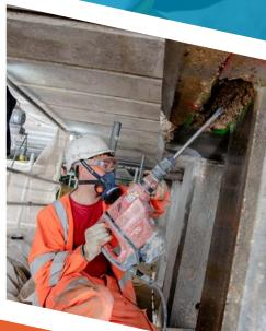
Marine structures suffer from deterioration due to corrosion of the steel reinforcement,
