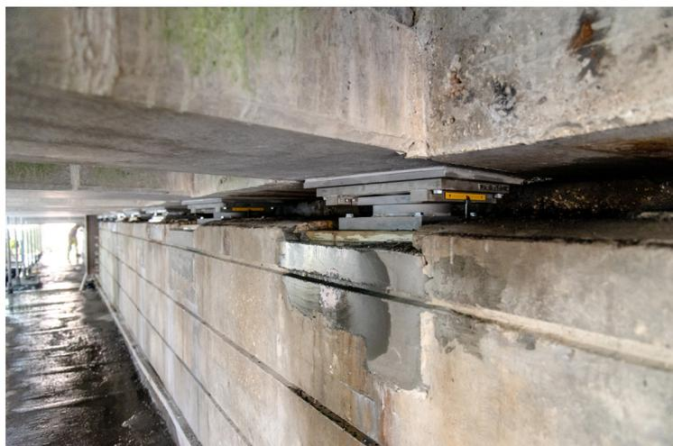
Initially CRL strengthened the structure to allow the bridge to be lifted. This involved infilling the service trenches that passed over the abutments to support the diaphragm sections.
