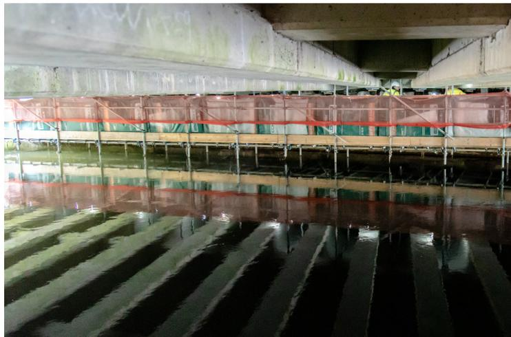
Following checking of the strength of these materials the bridge has been de-jacked on the north side with the gauges indicating the differential displacement between 0.25mm has been maintained.
