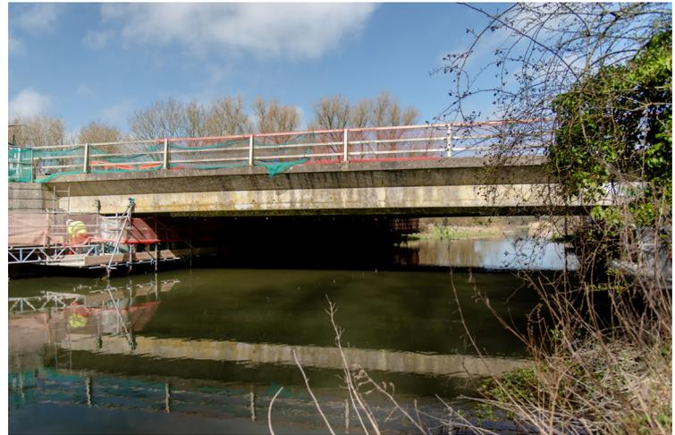
asphaltic plugs installed by Volker Laser. Concrete Repairs and anti-graffiti coating to the walkway abutment will complete the refurbishment to this bridge without adversely affecting the SSSI site.
