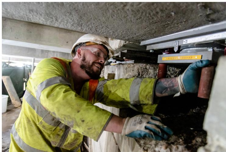
Following completion of a design and approved AIP jacks were installed either side of the bearings. With only a 20mm gap on the east side 60mm of the bearing shelf needed to be removed to allow the jacks to be installed without affecting the existing bearing supports.
